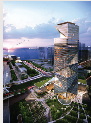
Songdo I-Tower (33 FL.)
